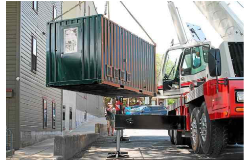
The kitchen of Farmers Hardware being put in place by a crane.
