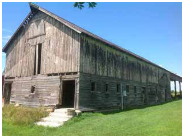
A crew from StoriedBoards reclaimed beech flooring from this circa-1930 barn on Durham Road in Stillwater, which builder Shawn Van Veghten then used while building a new house nearby. (Photo provided by StoriedBoards)
